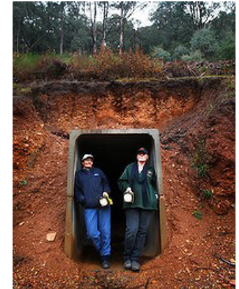
Some earth-covered bunkers built after previous fires remained in use and saved lives. Image: The Age 14/04/09.
