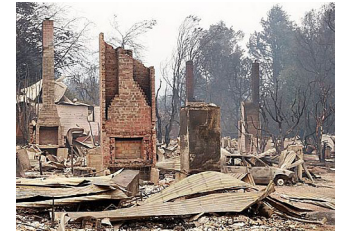
Masonry construction elements survived the enormous radiant heat and fire
