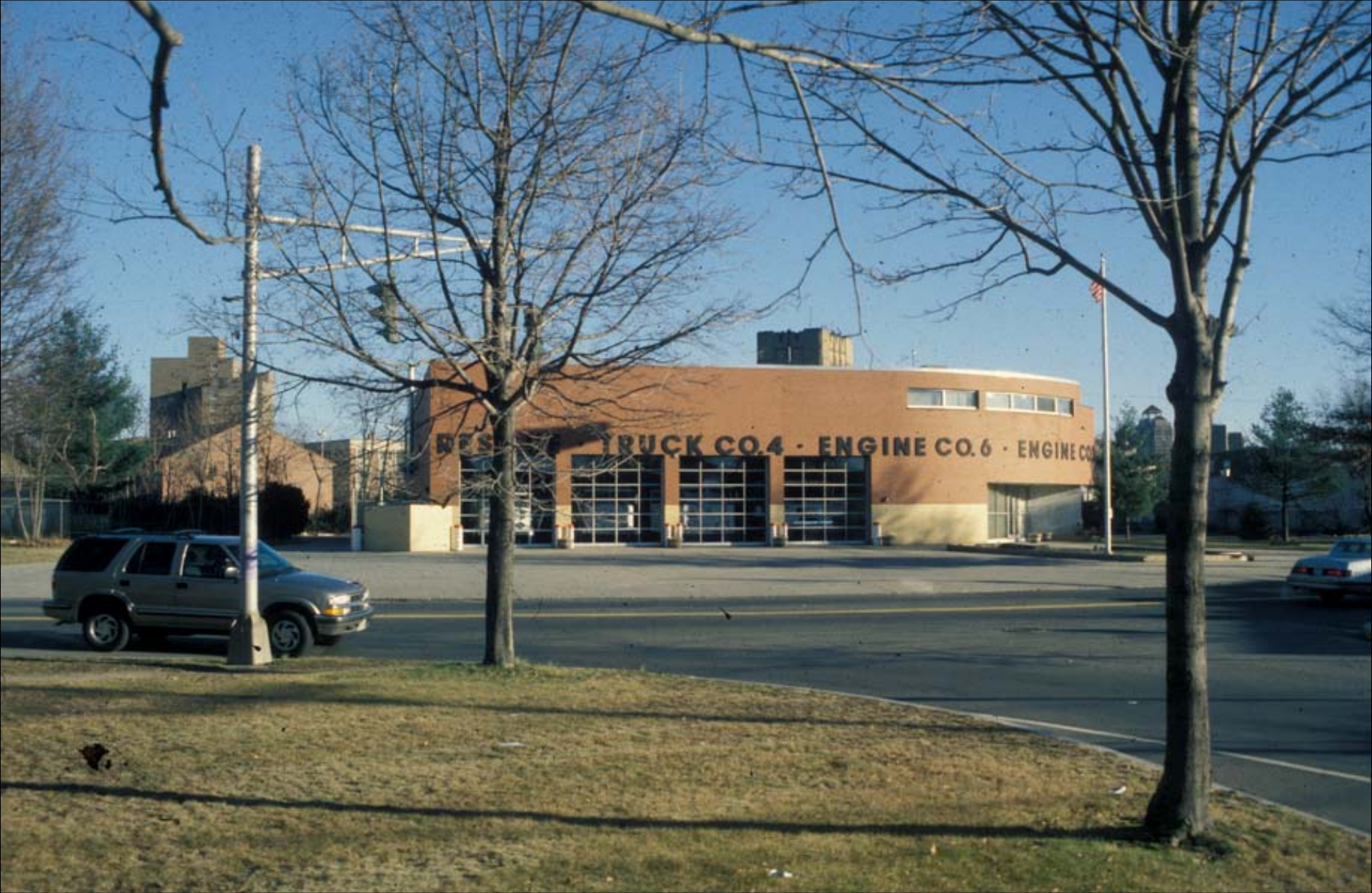
Dixwell Fire Station, New Haven 1974
