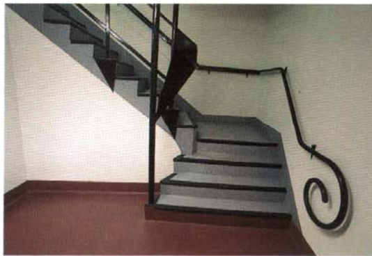
Figure 196 (see p. 123) Dandenong TAFE wing: stair handrail in Hair and Beauty section (photograph: John Gollings)
