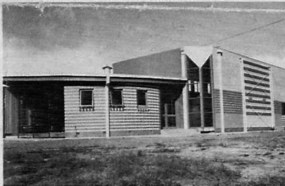
Resurrection School Hall Corrigan Road Keysborough Edmond & Corrigan 1979
